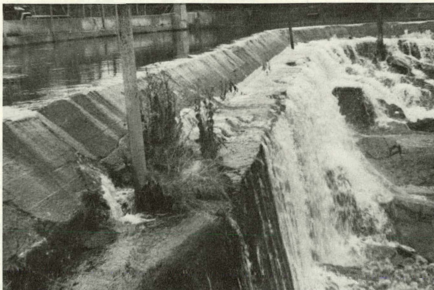
Huntington Falls Forebay leading to intake structure in upper right corner. Overflow due to surcharged reservoir. Note concrete condition near pole at left of picture.
