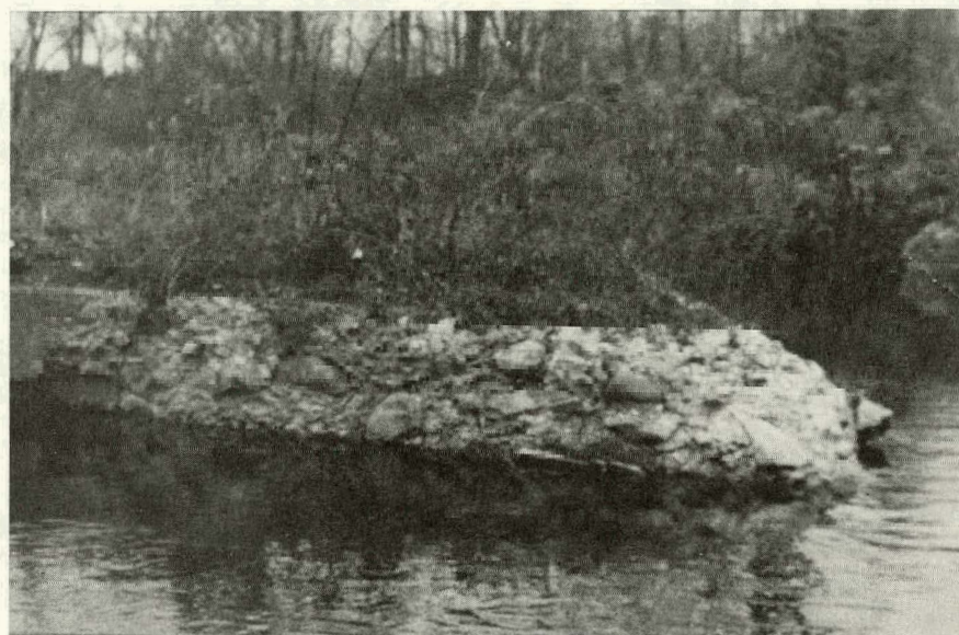
Huntington Falls entrance to Forebay showing concrete condition.
