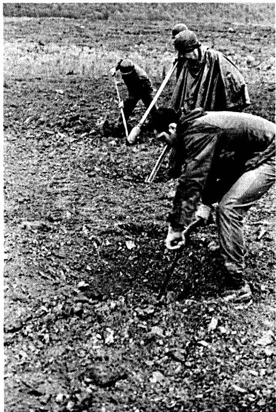
Figure A4. Posthole digger and hand auger being used to excavate slant holes of design G
