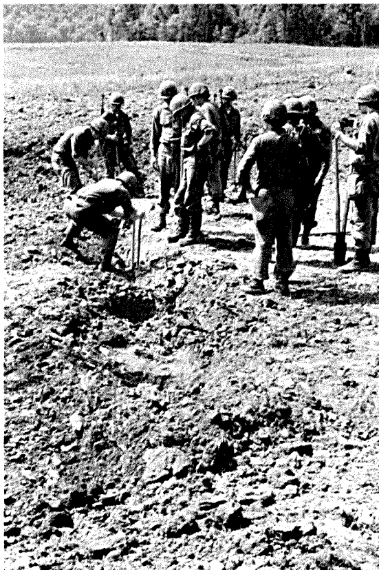
Figure A3. Posthole diggers being used to excavate emplacement holes
