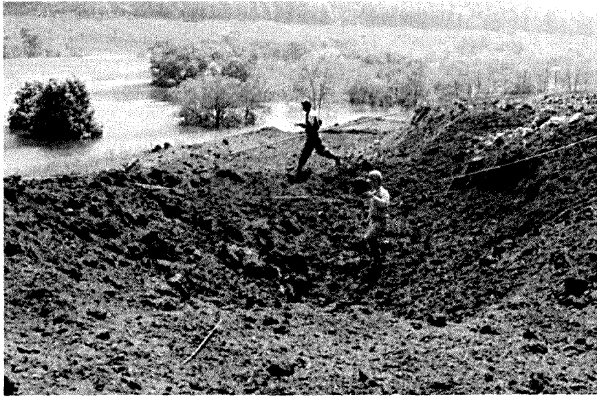
Figure 14. Design F3 fired at site II. This design was fired parallel to the road due to high uphill bank shown in photo
