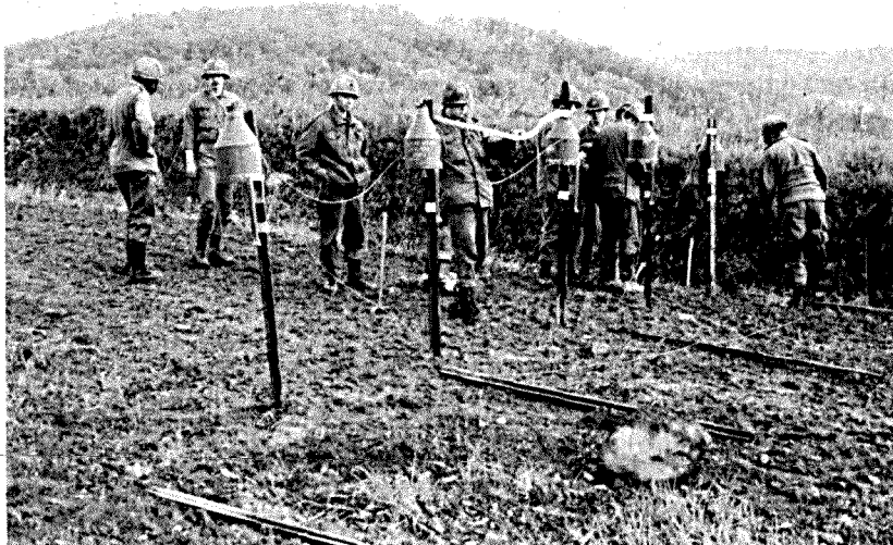
Figure A2. Shaped charges with metal pickets used to obtain 48-in. standoffs
