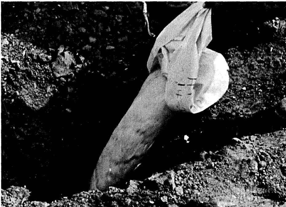
Figure 11. Slurry being poured downhole
