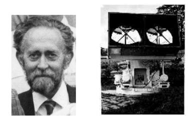
Figure 3. Left: Neil A. Porter (1930-2006) (Photo: D.J.Fegan) Right: The second ground-based gamma-ray telescope; the British-Irish experiment at Glencullen, Ireland c. 1964; the telescope consisted of two 90 cm searchlight mirrors on a Bofors gun mounting. The experiment was led by Jelley and Porter.
