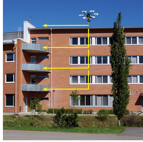
Figure 4. Yellow lines show flying heights of vertical scan measurement.
