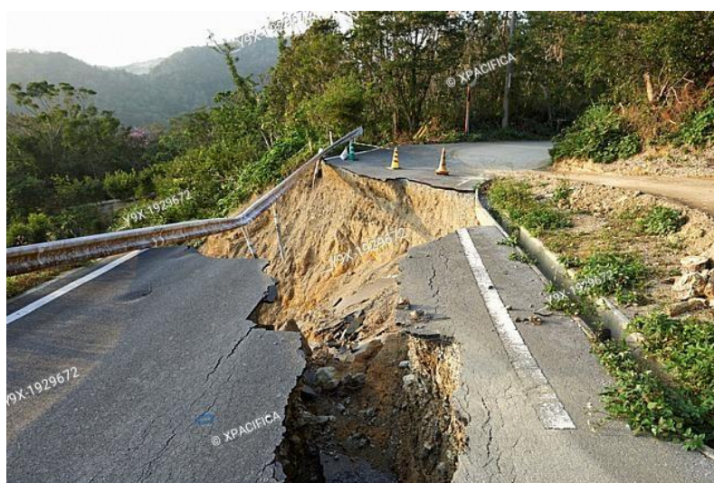
Figure 1: A landslide in a road located in a suburban area
