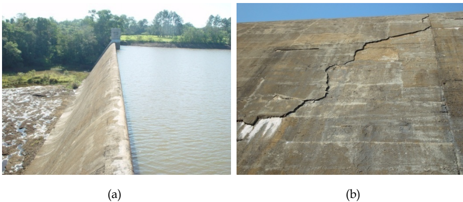
Fig. 8. (a) Overview of the spillway of the dam. (b) Detail of the displacement of the surface caused by hydraulic abrasive processes.
