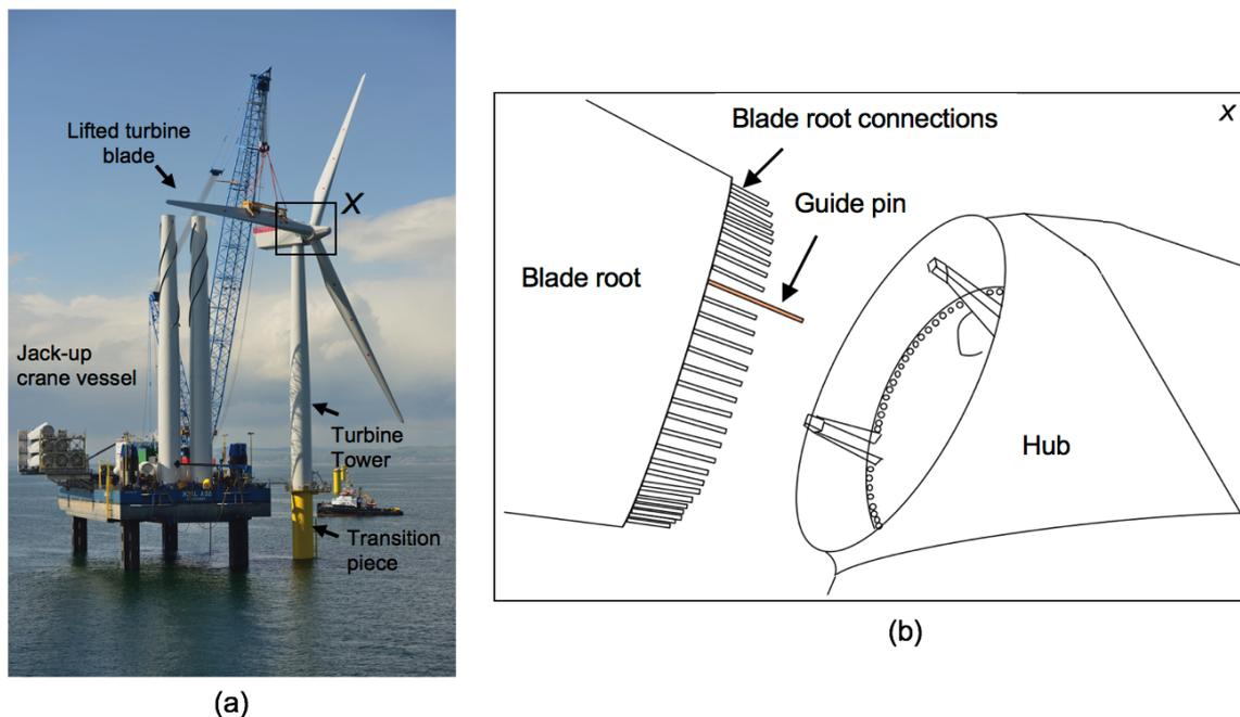
**Figure 2.** (a) Wind-turbine blade installation task using jack-up crane vessel [28]; (b) Magnified view of blade-root mating task [29].
