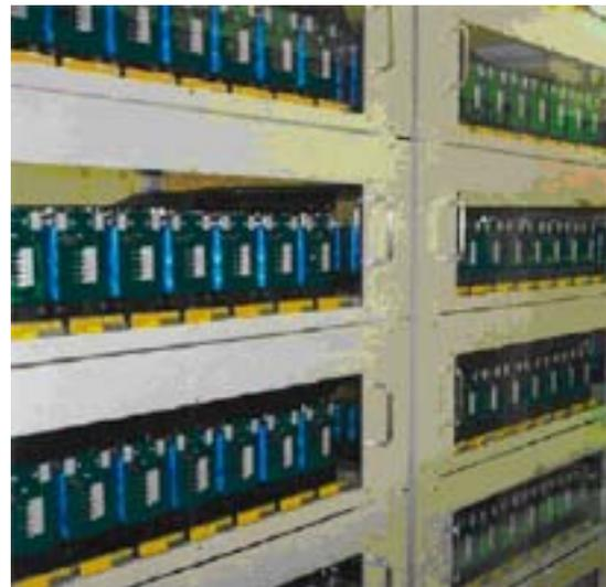
**Fig. 23. Large electrochemical capacitor storage system that provides short-time uninterruptible power.** (Photo courtesy of Nippon Chemi-Con)
