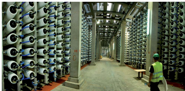
Fig. 1 Hadera RO Desalination Plant, Israel, 127 million m 3 year -1 . The Hadera seawater desalination plant in Israel, among the worlds most efficient, contains tens of thousands of RO membrane cartridges. Courtesy of IDE Technologies Ltd.
