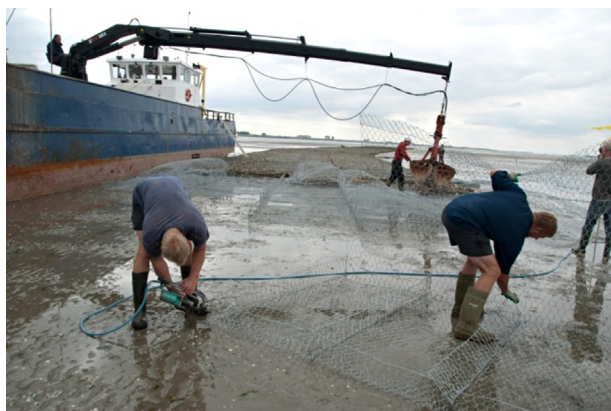
Fig. 15. Placement of gabions with oyster shells (courtesy: T. Ysebaert).
